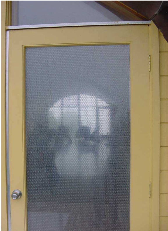
Fig 1. Visual performance of the bubble-glazed balcony door observed from outside. Interior details some 18m away are still recognizable. The bubbles have 10mm diameter and the bubble-wrap sheet is supported along the inside glass edges using aluminum channels.
