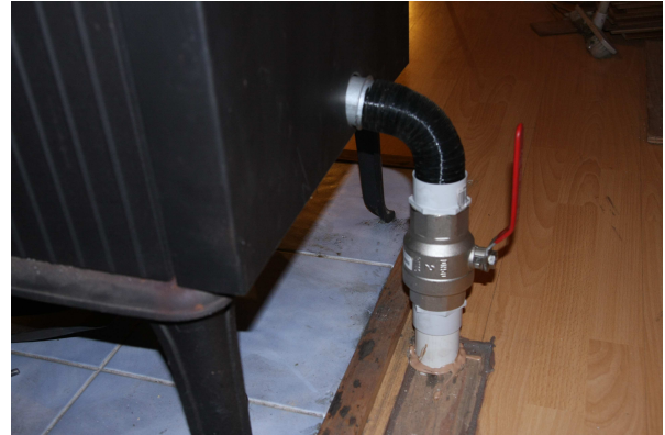
Fig 2. Flexible aluminum duct and ball valve at the back of the stove. Aluminum duct is cold to touch when the wood stove is hot.
